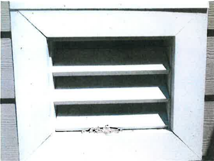
(TYPICAL) FLOOD VENT IN GARAGE WALL 3/29/2013
