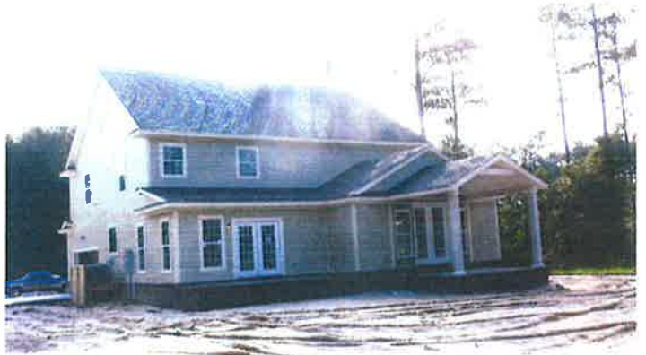
REAR VIEW/CONDENSING UNITS 08/26/2010
