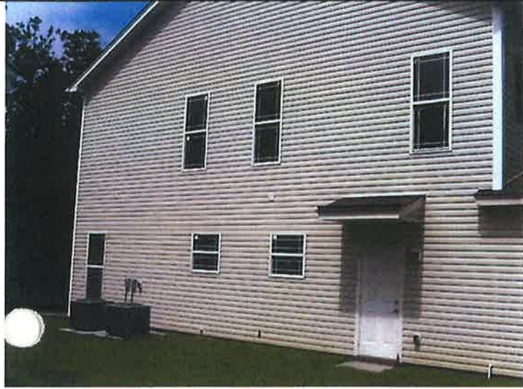
LEFT SIDE VIEW/AIR-CONDITIONING COMPRESSORS 06/18/2009
