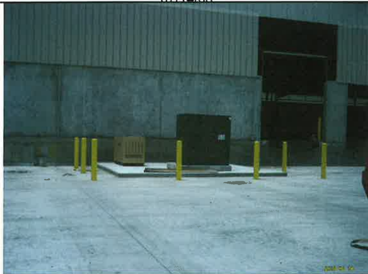
ELECTRICAL GENERATOR/TRANSFORMER PAD 07/14/08
