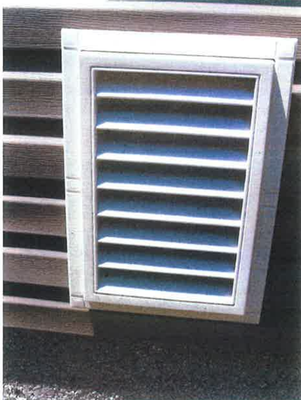
FLOOD OPENINGS (GABLE VENT/5 TOTAL) 04/23/2010
