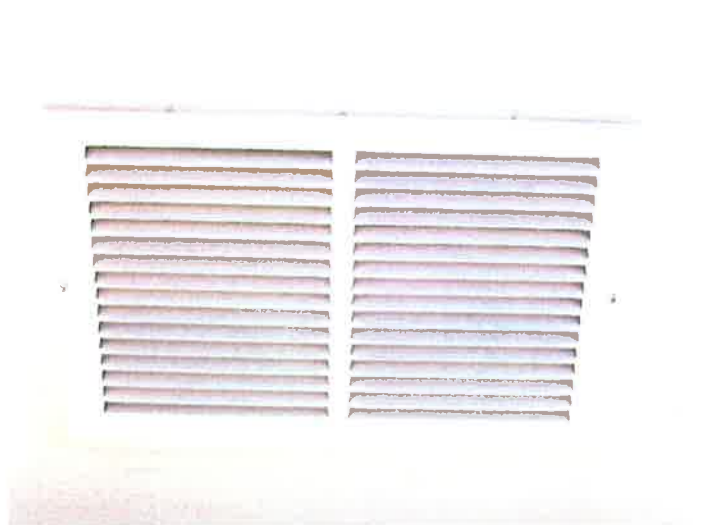
FLOOD OPENINGS IN DOOR (4 TOTAL) 4/23/2010
