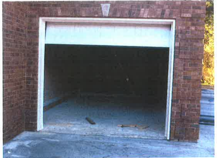
ENCLOSURE (GARAGE) VIEW 12/29/2009
