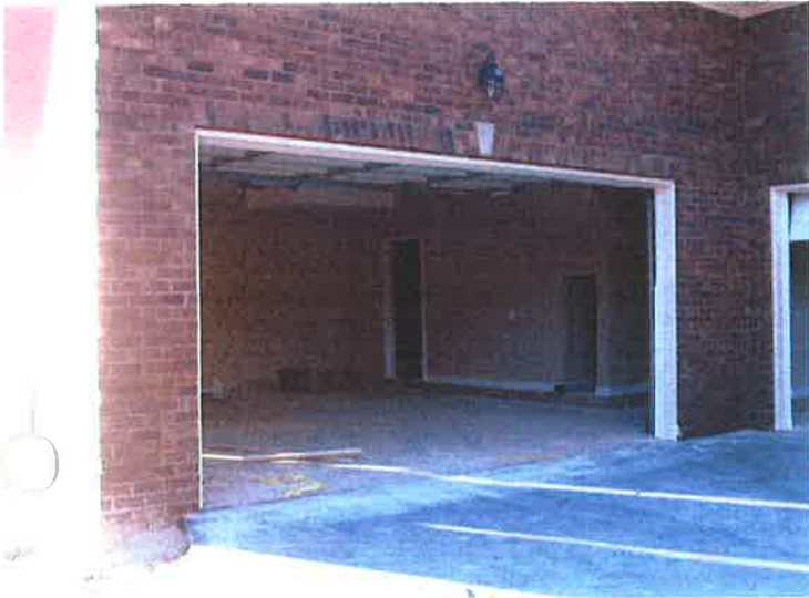
ENCLOSURE (GARAGE) VIEW 12/29/2009
