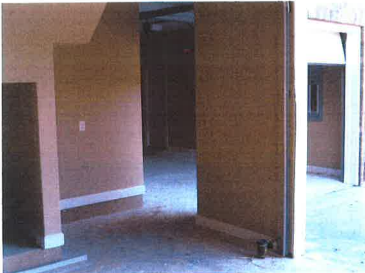
ENCLOSURE (GARAGE) VIEW 12/29/2009
