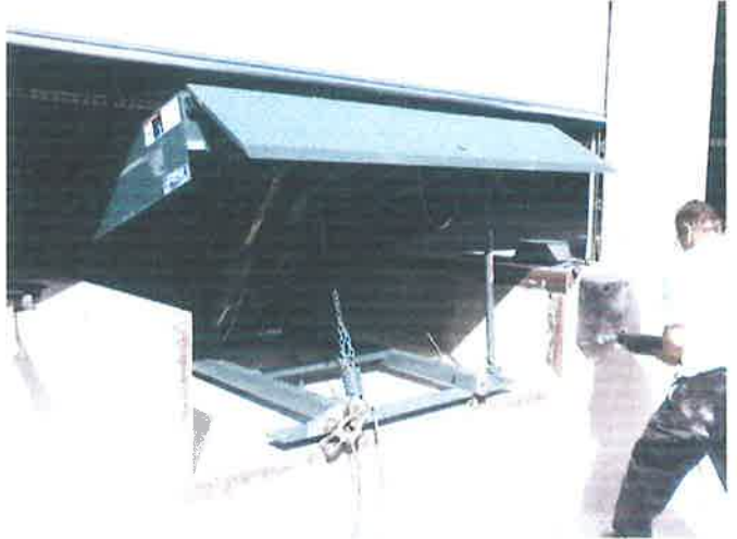
TYPICAL HYDRAULIC DOCK LEVELER & PIT 10/22/2009
