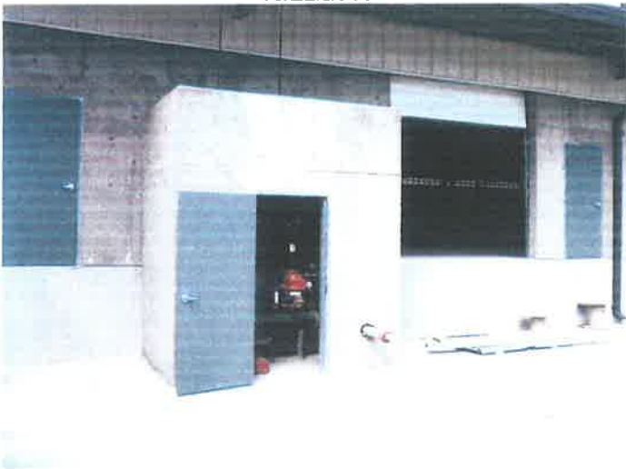
BOOSTER PUMP HOUSING 10/22/2009
