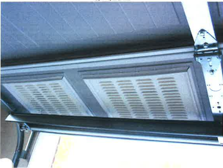
INTERIOR VIEW OF GARAGE DOOR FLOOD OPENINGS/VENTS OF BUILT-IN GARAGE 3/14/2012
