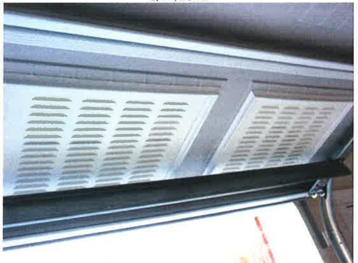
INTERIOR VIEW OF GARAGE DOOR FLOOD OPENINGS/VENTS OF BUILT-IN GARAGE 3/14/2012
