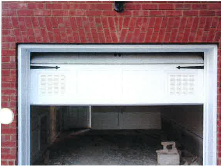
INTERIOR VIEW OF GARAGE DOOR FLOOD OPENINGS/VENTS OF BUILT-IN GARAGE 3/14/2012
