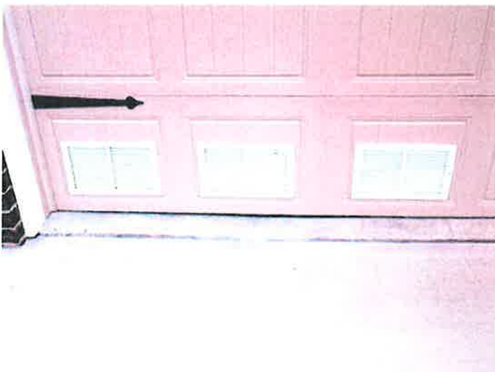
TYPICAL GARAGE DOOR FLOOD OPENINGS 09/18/2012
