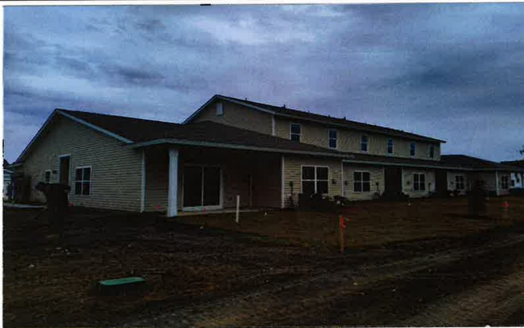
Photo Two Caption: REAR RIGHT VIEW 11/20/2023
