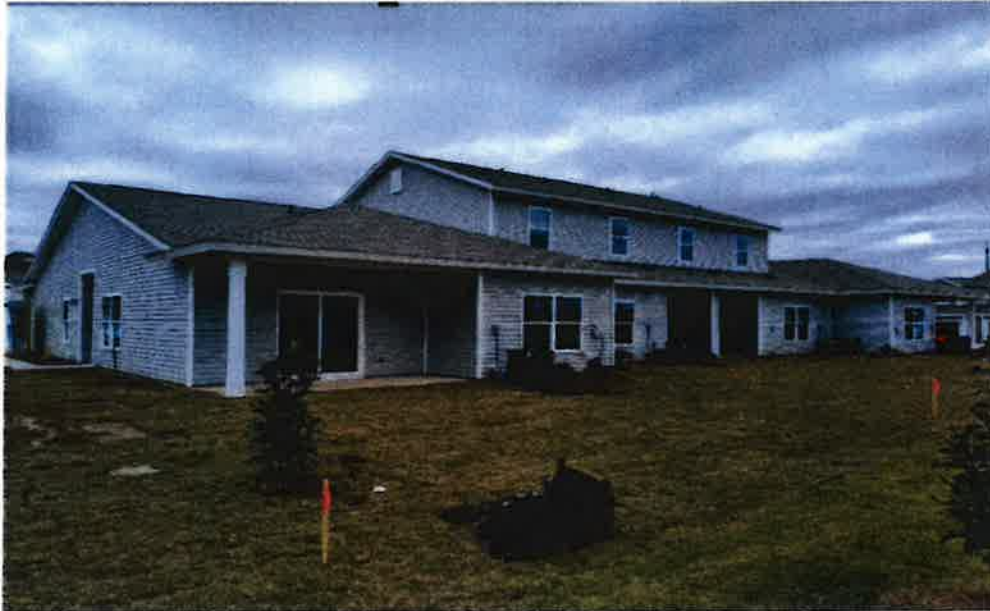
Photo Two Caption: REAR RIGHT VIEW 11/20/2023
