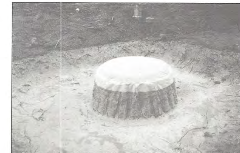
Figure 6-28.7 Equivalent Inlet Sediment Trap
