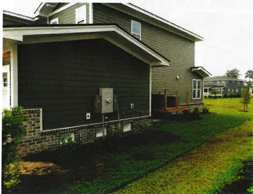
Flood Vents and HVAC (7/23/2025)
