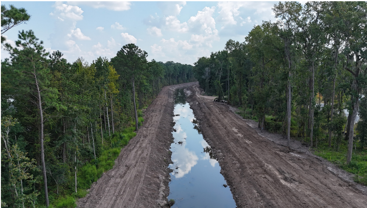
Pipemakers Canal Widened by 40 feet
